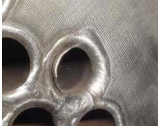
Figure 36. Partially TIG welded the sleeve to the 7' long sleeves into the parent stainless steel tubes.
