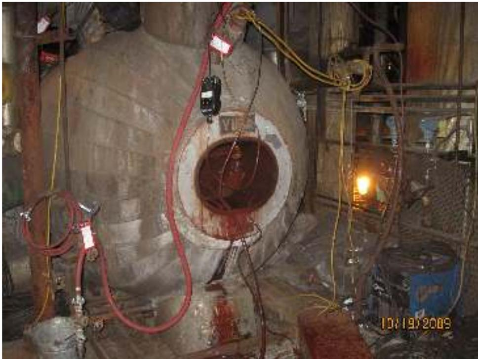
**Figure 2 Supercritical HP Feedwater Heater 7W Hemi-head with 14"X18" Man Way**
