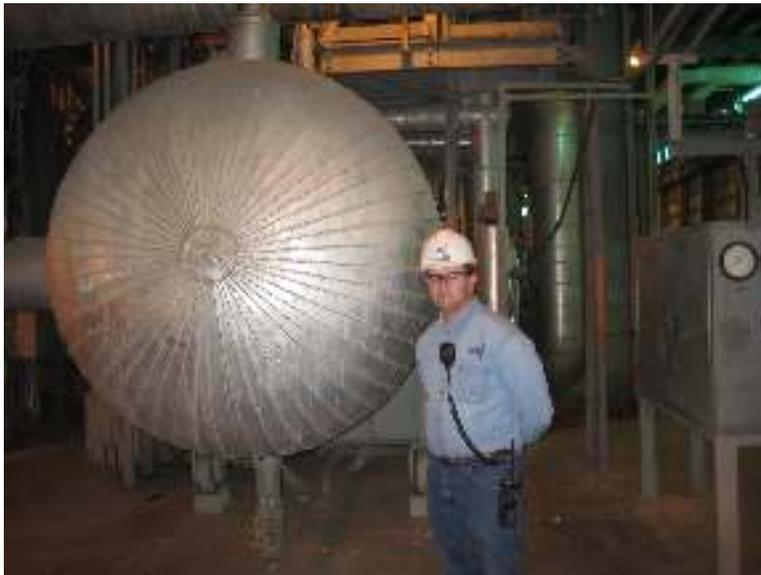
**Figure 2. One of Two IP FWH's with (1,134) 3/4"OD x .035" SA-688 304 SS U-tubes.**
