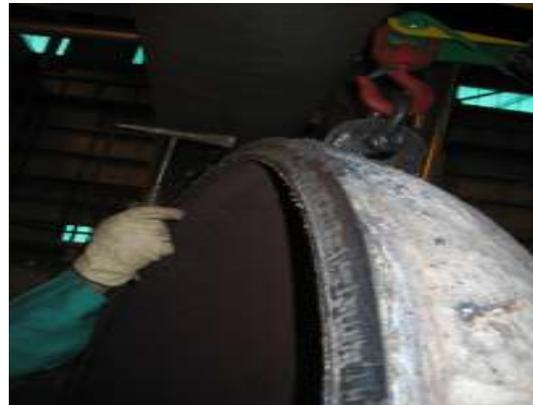
**Figure 11. Shell cut prepped for re-welding.    Figure 12. Head Cut provides weld prep.**
