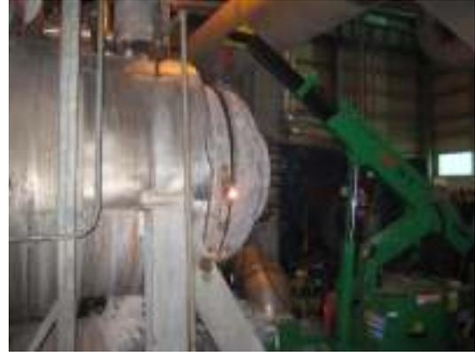
**Figure 9. Cutting shell with track cutter    Figure 10. Cut head with rotary torch cutter**
