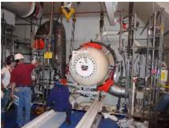
Fig 7. Condenser neck heater prior to removal.
